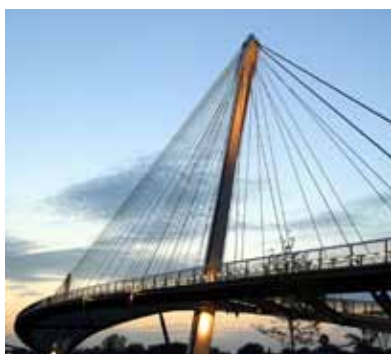
The Passerelle des Deux Rives footbridge, where the heads of State and government of the NATO countries will be welcomed
